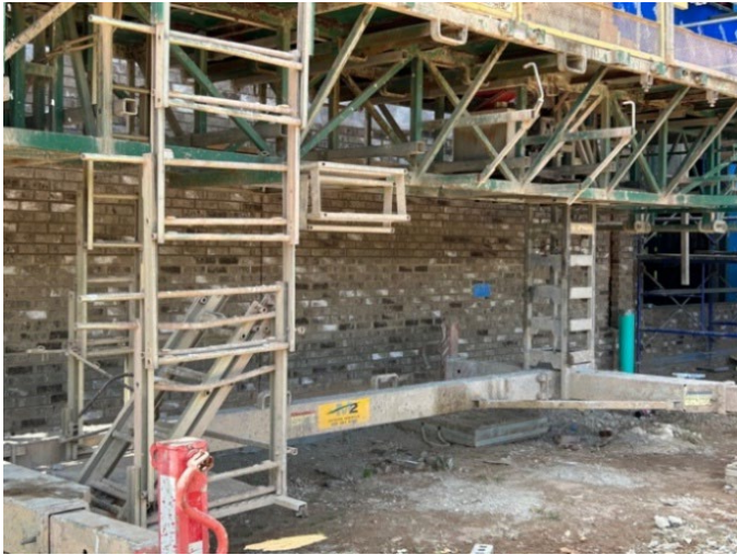
Brickwork on the south side of the building
